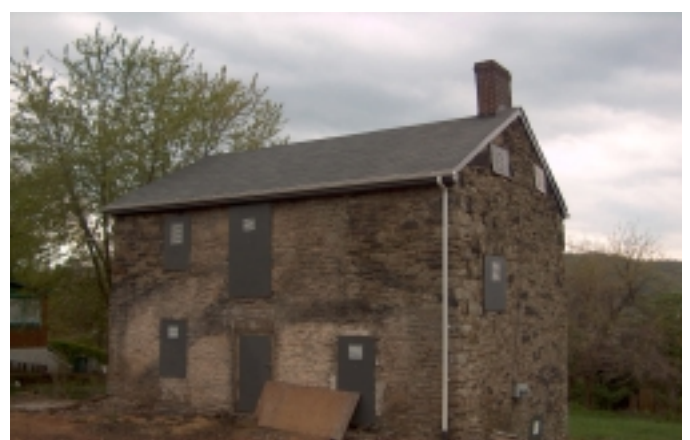
The Hazelwood Initiative stabilized the John Woods House
