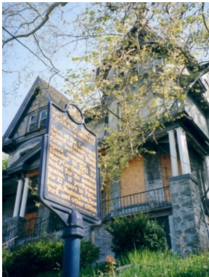
The PHMC historical marker outside the National Negro Opera Company home can be misleading. The house is not a protected city landmark.
