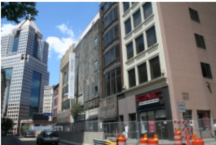
The next victims: These historic buildings Downtown are being demolished.
