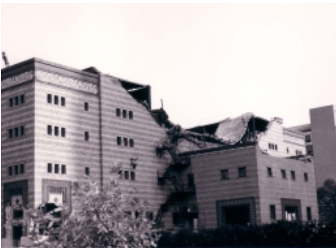
Syria Mosque being demolished in 1991.
