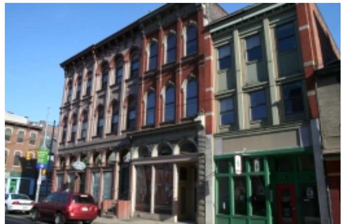
East Carson Street was one of the first Main Street programs in the U.S.
