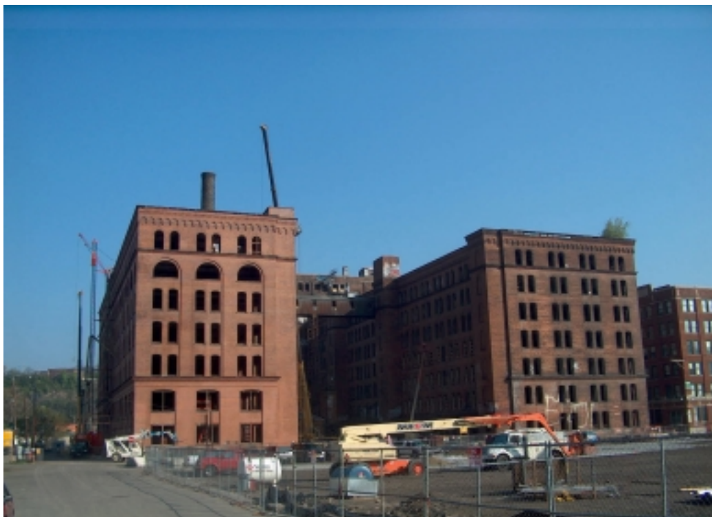
The Armstrong Cork Factory is listed on the National Register of Historic Places, has a preservation easement, but is not a city-designated historic landmark.
