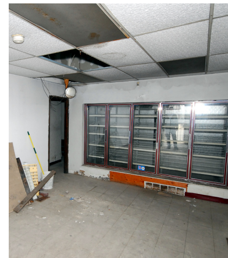
1727 Bedford (Front) - Storefront interior
