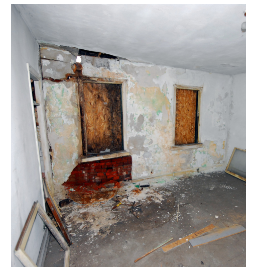
1727 Bedford (Rear) - 2nd floor bedroom
