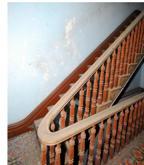
1727 Bedford (Front) - Stairwell
