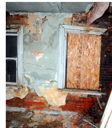
1727 Bedford (Rear) - 2nd floor bedroom
