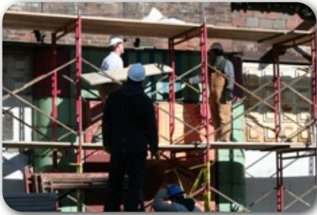
Renovation of the New Granada Theatre in the Hill District
