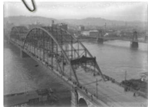
The third Sixth Street Bridge (1892-1927)
