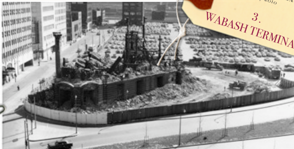
Demolition of the Wabash Terminal in 1955
