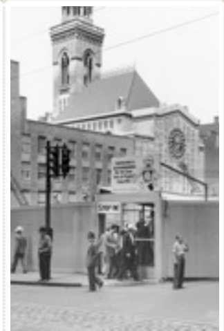
Construction of Alcoa Tower, 1950
