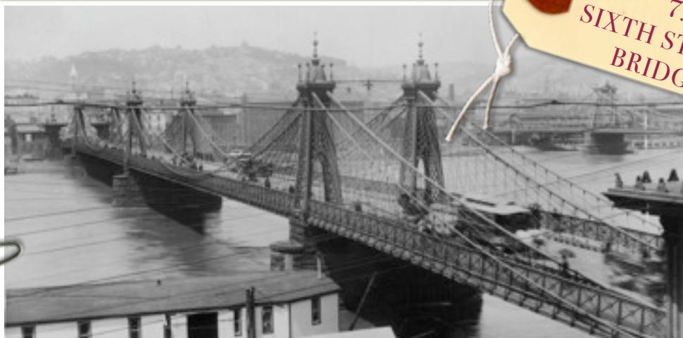
Roebling's Sixth Street Bridge (1859-1892)
