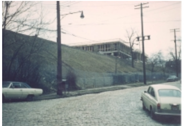
After: The same site after demolition. Fall 1970.
