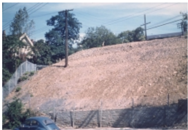
After: The same site after demolition. September 1970.
