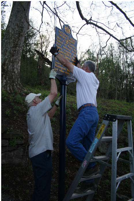
Installation of new replacement PHMC marker, May 2, 2007. Photo: Dan Holland
